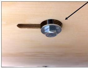
2. Remove the ceiling mounting plate by loosening the bolts enough so that you can slide it left or right. Slide until the bolts and washers align with the circular aperture (right), then lift the mounting plate off the Ceiling Shower.
